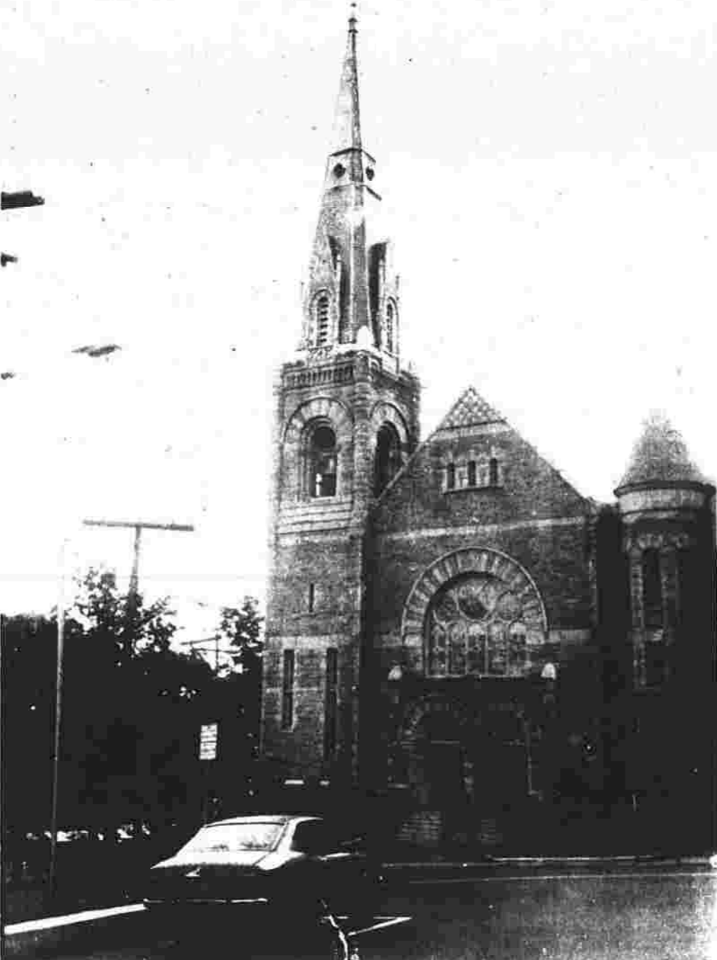
Church at dusk The stately Union Congregational Church in Rockville, forms a stately silhouette on the Skyline at dusk. The church recently underwent extensive renovations after it was severely damaged by a fire. (Herald photo by Richmond)
